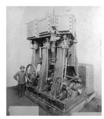
Steam engine for the Tatsutagawamaru cargopassenger ship, manufactured in 1894 (3 cylinders, 65 hp)
