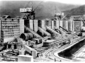
Installation of penstocks (built in 1944) during construction of the Songhua River Power Station (Manchuria)
