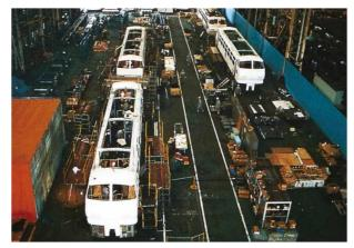
Electric locomotive manufacturing line at Sakaide Works (1989)
